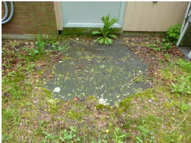
Worn asphalt paving at walks and front and rear stoops is shown to be replaced in Year 1.
