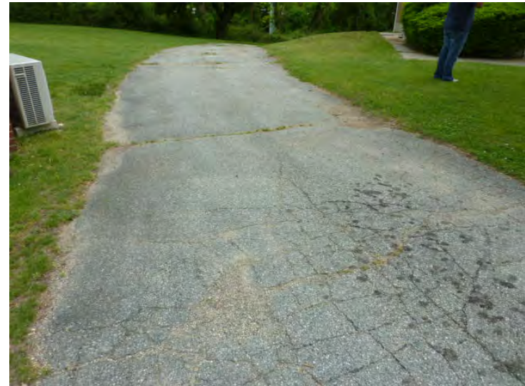
Typical cracking and sub-base failure at garage drives.
