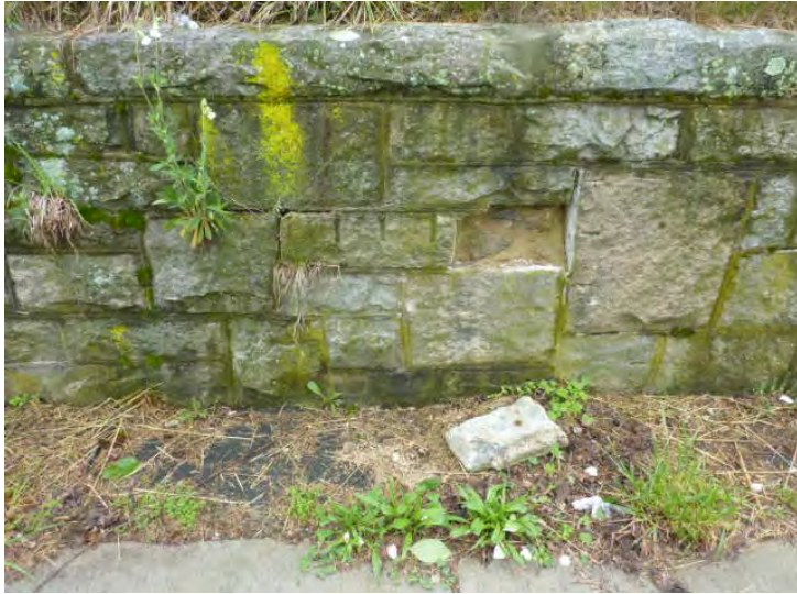
Typical distress and failure at Riozzi Court of the mortar set stone retaining walls along Colman Street and Garfield Avenue and the dry set stone retaining wall along the southeast property line.
