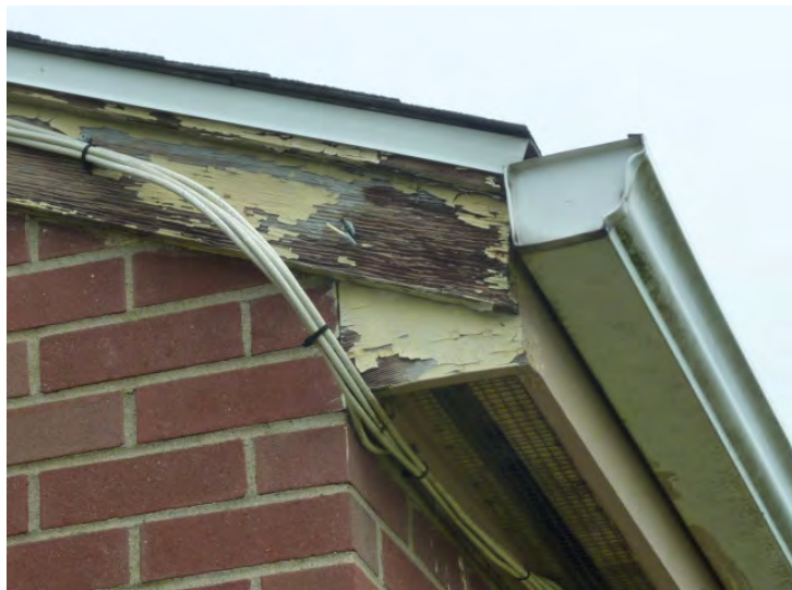
Typical failures at wood fascia and trim.
