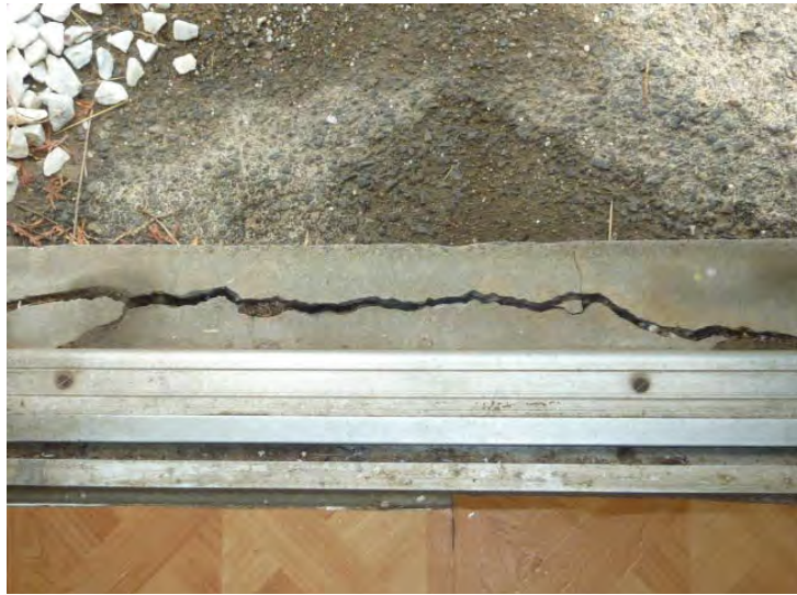
Typical cracked door sills at select locations are shown to be repaired in Year 1.
