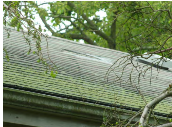
Organic growth and storm damage at shingled roofs will be repaired by maintenance. Roofs are 20 years old and are shown to be replaced in Year 5 based on condition.
