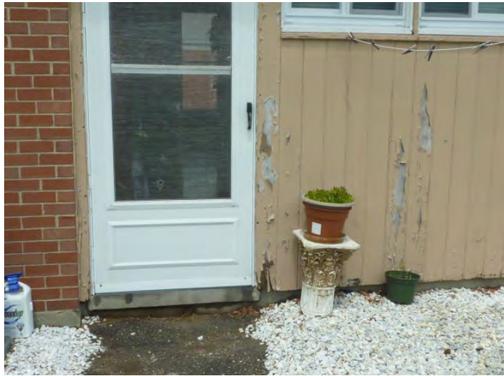
Typical rotted door trim and paint failure at all buildings.
