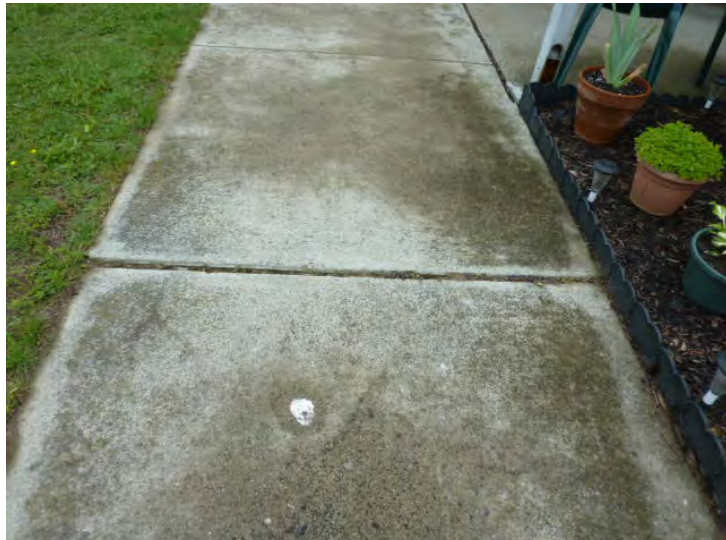
Typical trip hazard and worn concrete walks. Elimination of trip hazards and replacement of concrete walks is shown in Year 1.
