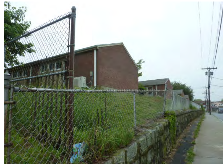
Rusted chain link fence and failing mortar set stone retaining wall along Garfield Street at Riozzi Court are shown to be replaced in Year 1.
