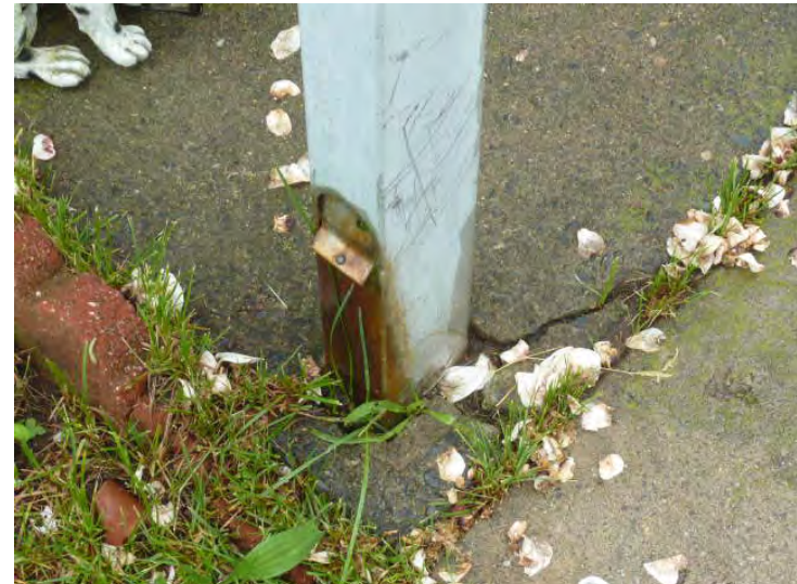
Rusting roof post anchors are causing concrete failures at post bases at select locations.
