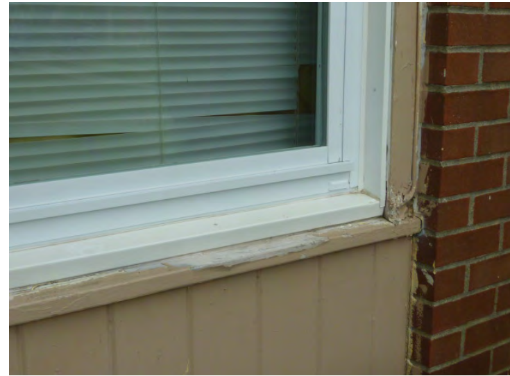
New windows were installed over rotted wood substrates and are shown to be repaired and re-caulked over the plan and replaced in Year 20 based on condition.
